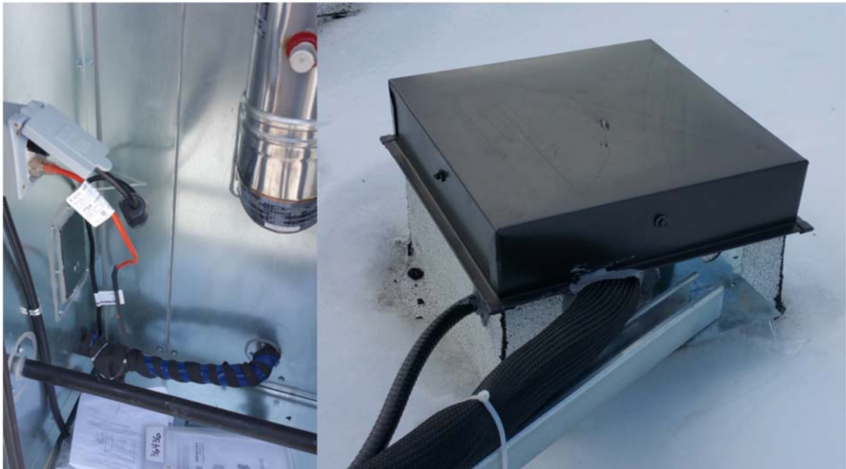
Image 2: Freeze protection system
