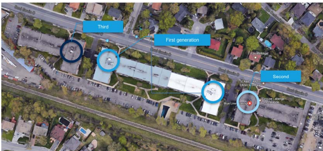
Image 4: Location of make-up air units on the Le Lalande building
