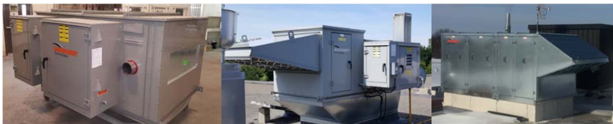
Image 1: First, second and third generation (condensing) make-up air units (shown from left to right)
