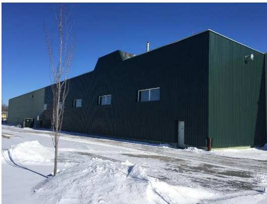
Cascades's solar wall in Candiac's plant.
