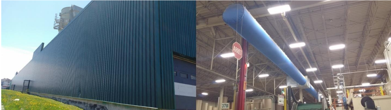
Cascades's solar wall in Vaudreuil's plant.
